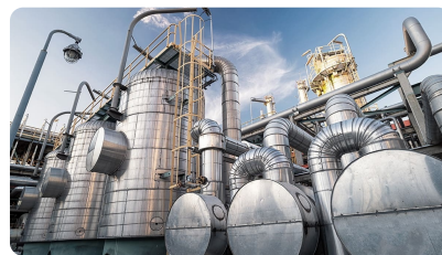
Chemical and Process Technology - Aerzen
